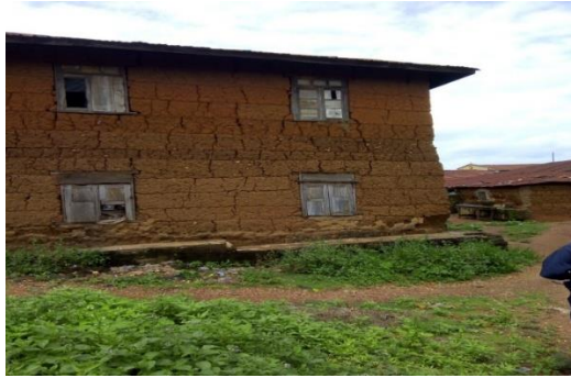
Figure 1: Storey Building with Pitched Roofs and Substantial Overhangs and Thick Earthen Walls Providing Thermal Mass (Omoniyi, 2018)
