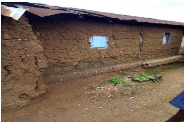
Figure 2. Building with Wooden Windows with Eroded Foundation (Omoniyi, 2018)
