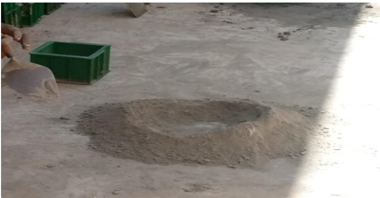
Figure 2. Photo graph of the Mixing process of Concrete
