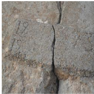
Figure 1. Concrete of the Oued Fodda dam (Orleans-Ville, Algeria)
